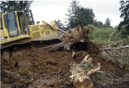
Bulldozer forming windthrow mounds on a restoration project
