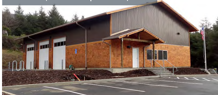
Arch Cape Station | Arch Cape, OR
