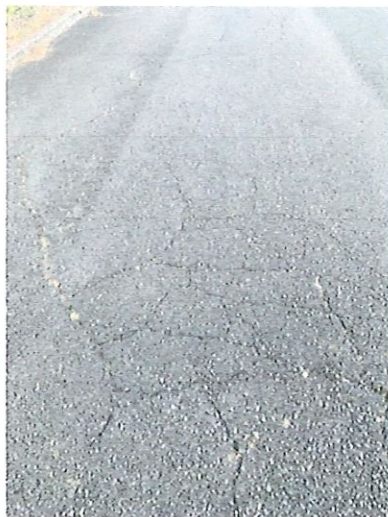
3. More pictures of lower portion of road where water runoff has eroded under pavement and has caused sinkage of concrete easily visible of shifting ground.
