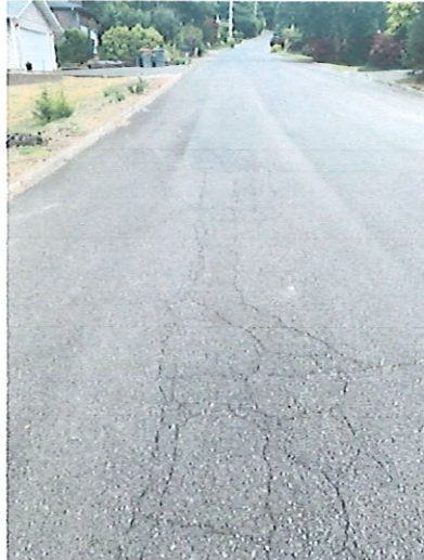
3. More pictures of lower portion of road where water runoff has eroded under pavement and has caused sinkage of concrete easily visible of shifting ground.
