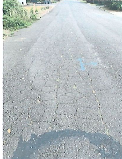
3. More pictures of lower portion of road where water runoff has eroded under pavement and has caused sinkage of concrete easily visible of shifting ground.
