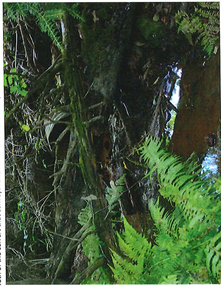
outh of the culvert that conveys runoff from the catch basin pictured above.
