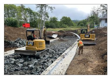
Coho Creek is a tributary to Neawanna Creek that had run through a 36-inch corrugated steel culvert under S. Wahanna. The culvert and two additional degraded and partially blocked culverts immediately upstream are being removed and replaced. A 19-foot bottomless arch culvert is being installed beneath S. Wahanna, which will help control flooding within the local waterways and enhance passage of native fish, including coho, Chinook, chum, Pacific lamprey, winter steelhead and cutthroat trout.
